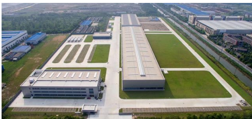
In May 2018, the TRUMPF subsidiary JFY in Yangzhou opened the Group's largest production site worldwide to date. The production area is 19,000 m 2 .
