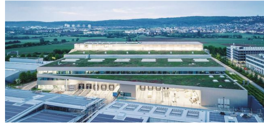
<p>Power from the rooftops: TRUMPF is steadily expanding its in-house generation of renewable energy through sources such as large photovoltaic systems.</p>
