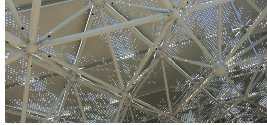
For the SoFi, A. Zahner used three TRUMPF machines to cut and punch 37,000 different panels with around 30 million irregularly distributed holes. (Source: © A. ZAHNER COMPANY)
