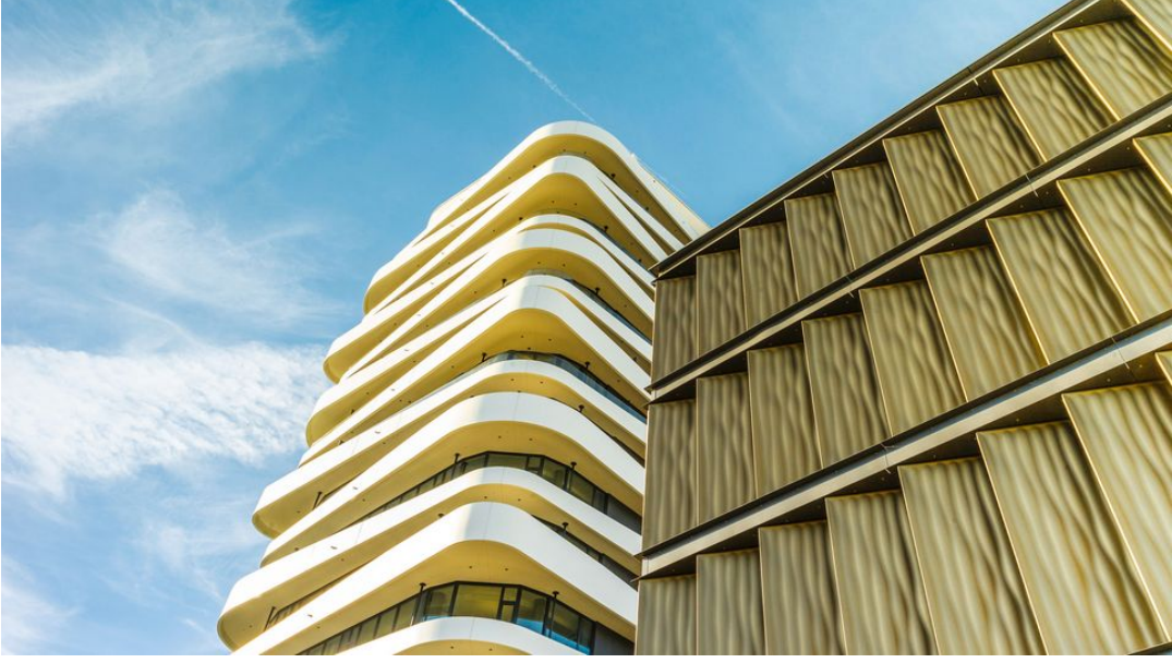
Multistory parking garage in Bietigheim-Bissingen (Source: TRUMPF)
