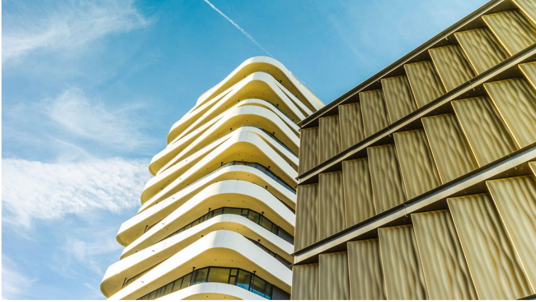
Multistory parking garage in Bietigheim-Bissingen (Source: TRUMPF)
