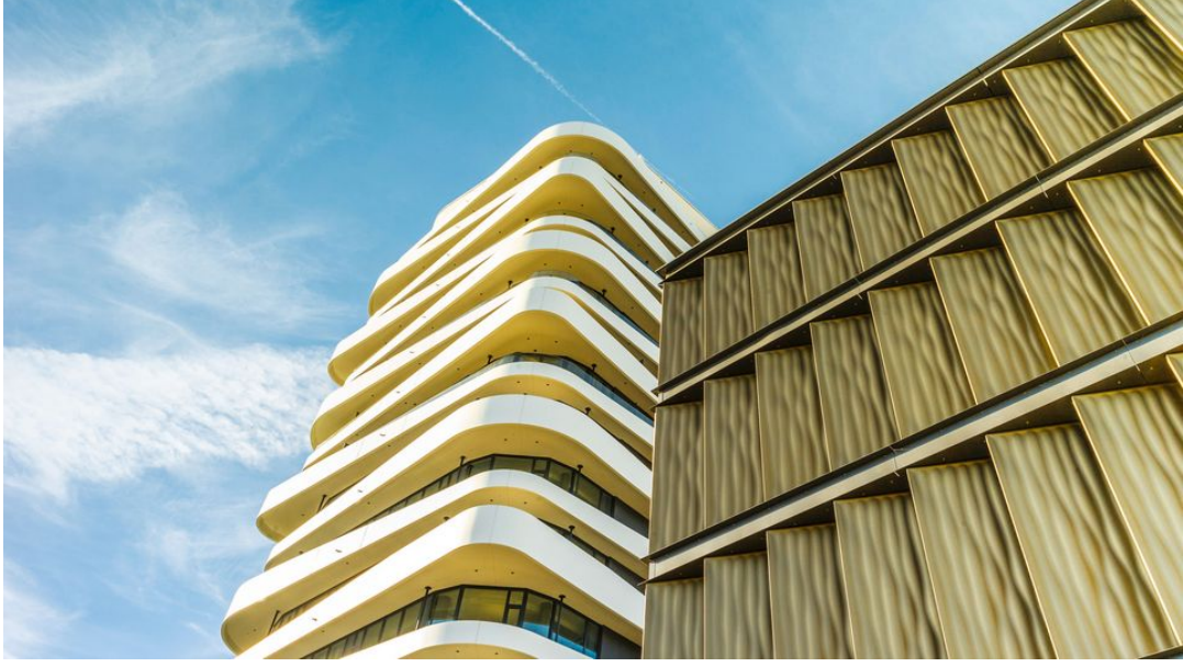
Multistory parking garage in Bietigheim-Bissingen (Source: TRUMPF)
