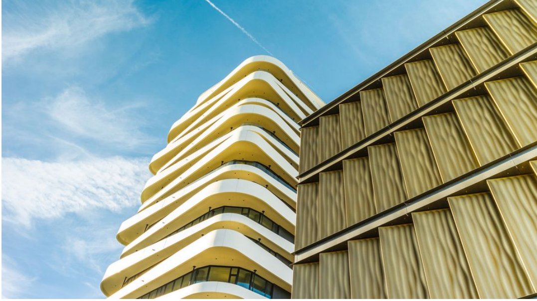
Multistory parking garage in Bietigheim-Bissingen (Source: TRUMPF)
