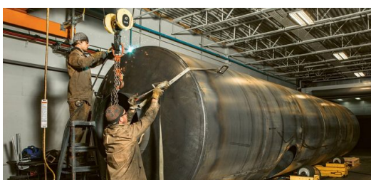
As a second-generation owner, CEO Casey D. Osborn is determined to keep the company strong despite its relative isolation – and that means embracing diversification. “Our core business – compression systems for natural gas plants – experiences significant fluctuations,” he says.
