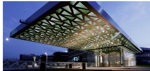
In 2016, the Ditzingen Campus won the Industry Prize in the category "Urban Planning Facilities". Shown above: The gatehouse.
