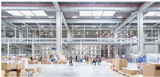
The new TRUMPF logistics center has a surface area of 13,000 square meters, a ceiling height of 18 meters, and delivers more than 60,000 stock items per month.
