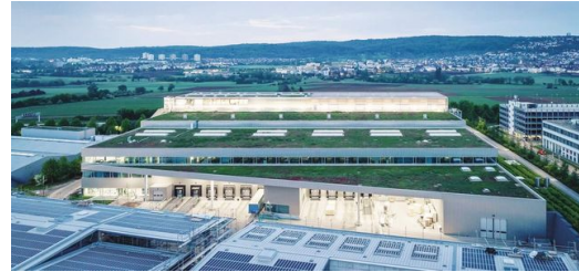
Power from the rooftops: TRUMPF is steadily expanding its in-house generation of renewable energy through sources such as large photovoltaic systems.
