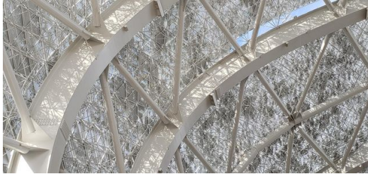
The perforated panels allow light and air to pass through - it was the architects' ambition to build an open arena in which people are nevertheless protected. (Source: © A. ZAHNER COMPANY)
