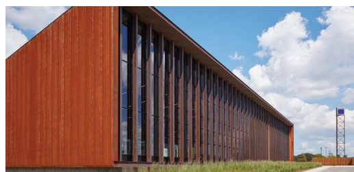
The building links the history of the "Rust Belt" as the oldest and largest industrial region in the USA with high-tech digitally connected production. Picture: Steve Hall © Hall+Merrick
