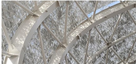
The perforated panels allow light and air to pass through - it was the architects' ambition to build an open arena in which people are nevertheless protected. (Source: © A. ZAHNER COMPANY)
