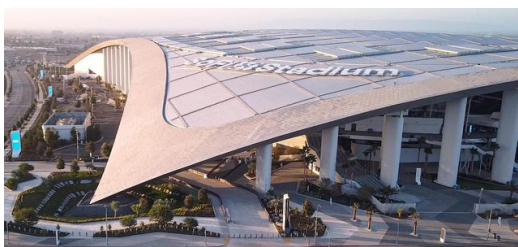
The roof of the SoFi Stadium is light and elegant. The cover made of the translucent plastic ETFE can be opened and closed. (Source: JESSE PACHECO, ARKO | © A. ZAHNER COMPANY)
