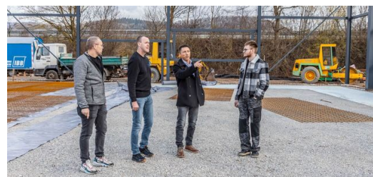
DELO is planning on relocating to neighboring Hechingen in September 2023. Construction work is in full swing. With a developed area of 2,000
