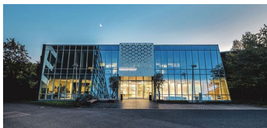
<p>Customer center: TRUMPF impresses customers with its combination of outstanding industrial architecture and superb product quality.</p>
