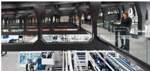
A bird's-eye view of the factory reveals a catwalk, the so-called "Skywalk": Spanning the full length of the 55-meter-long hall, with its material and information flow, it emphasizes the fact that the production facilities constitute a single, overall system. Picture: Steve Hall © Hall+Merrick
