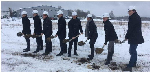
<p>The ground-breaking ceremony for the new production hall at the TRUMPF site in Hettingen in January 2019. 120 employees are to move into the competence center in two years.</p>
