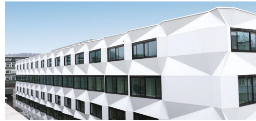
As painted: The facade of the University of Lucerne comes from BIGSTEEL. (Picture: Niels Schubert)
