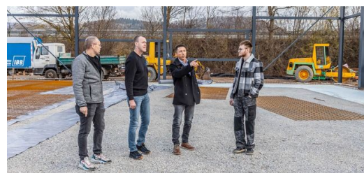
DELO is planning on relocating to neighboring Hechingen in September 2023. Construction work is in full swing. With a developed area of 2,000 square meters, he is aiming to more than double production compared to
