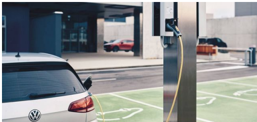
Sustainable development – the charging stations for the company's vehicle fleet are powered by rooftop solar panels.
