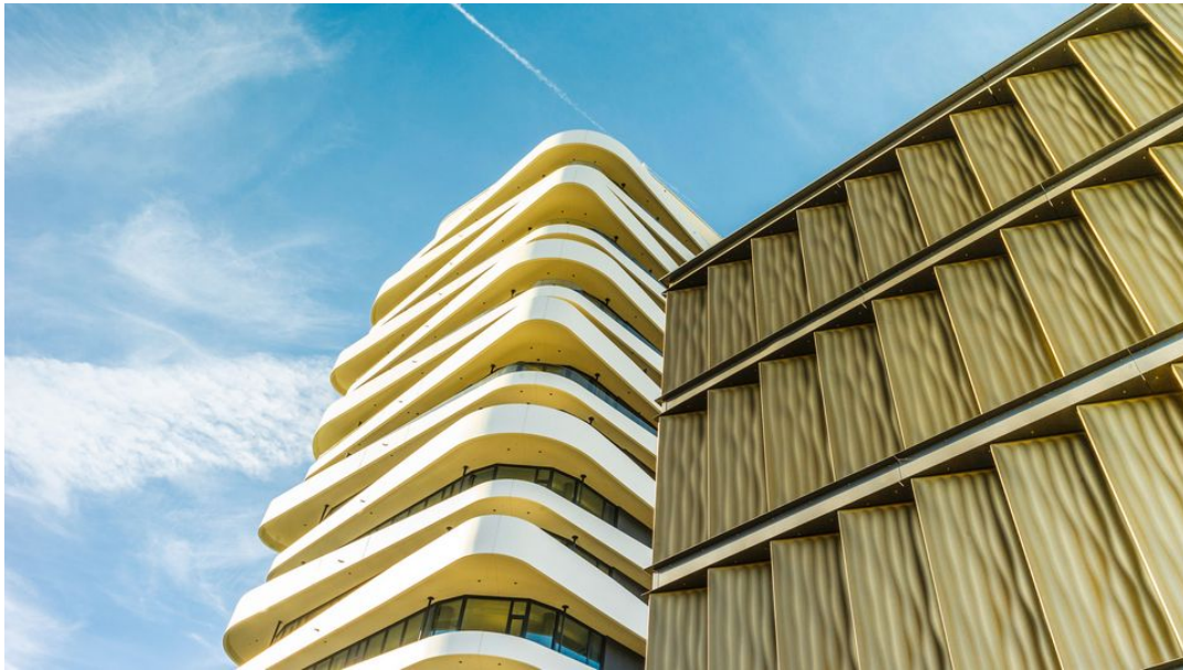
Multistory parking garage in Bietigheim-Bissingen (Source: TRUMPF)
