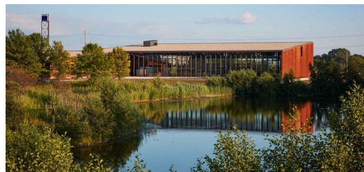
In Chicago, TRUMPF inaugurated a Smart Factory for networked sheet metal processing in 2017.
