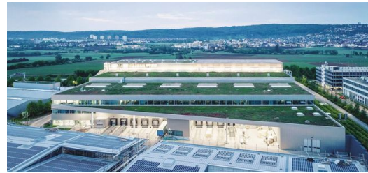
Power from the rooftops: TRUMPF is steadily expanding its in-house generation of renewable energy through sources such as large photovoltaic systems.
