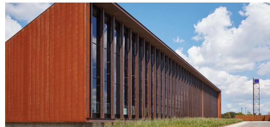
The building links the history of the "Rust Belt" as the oldest and largest industrial region in the USA with high-tech digitally connected production. Picture: Steve Hall © Hall+Merrick
