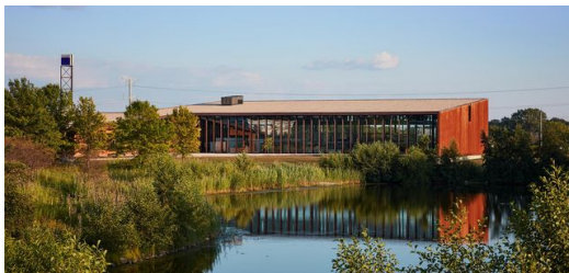
Chicago was consciously chosen as the location for the Smart Factory. The directly adjacent states contain around 40 percent of the country's entire sheet metal working industry. Picture: Steve Hall © Hall+Merrick
